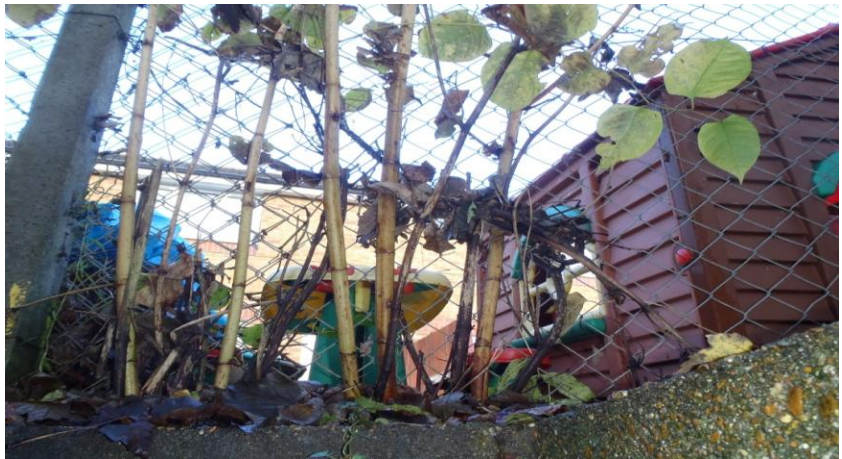
Knotweed growing through joints in concrete retaining wall on Lukely Brook, IoW
