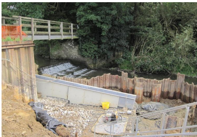
Arun Fish pass during construction
