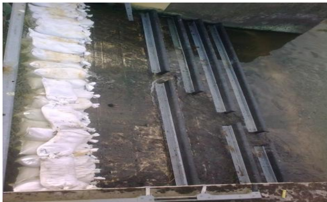
Low Cost Baffle during installation
